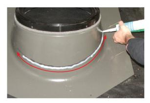
**5** Apply a generous bead of silicone along the bottom of the marked line all the way around the perimeter of the standard flashing.
