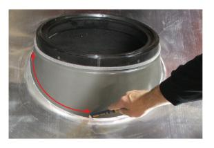
4 Mark the top perimeter of the tile flashing on the standard flashing. Then remove tile flashing.
