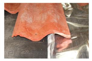
Caution should be taken not to penetrate the flashing with the tile fasteners.
