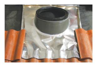
14 Start installing the tiles around the tile flashing system.
