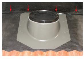
2 Overlap the top of the standard flashing with the base roofing material or underlayment to allow for proper drainage.
