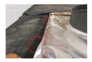
Create water diverters on the sides, by folding  $1^1/_2$ " of the flashing up on each side.
