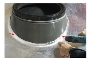
7 The screw holes should be pre-drilled perpendicular to the tile flashing surface and evenly spaced around the parameter of the tile flashing. Pre-drill holes with a 3/32" drill bit a 1/4" down from the top edge of the tile flashing. The 22" flashings should use all six screws, the 14" flashing should use five screws, and the 10" flashing should use four screws to fasten the tile flashing to the standard flashing.
