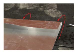
Oreate a water diverting channel by folding 3" to 4" of the tile flashing top edge over the tile flashing piece so that it runs parallel.
