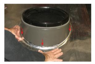
6 Reposition the aluminum tile flashing sheet over the standard flashing so you can barely see the line you marked.
