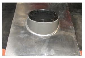
3 Place the aluminum tile flashing over the standard flashing. The top of the tile flashing should rest on the top of the standard flashing. The bottom edge should be positioned over the tiles.
