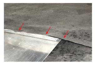
n Position the base roofing material or felt over the folded top edge of the tile flashing, stopping short of the vertical fold.
