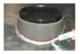
Once secured, provide another bead of silicone over the joint between the standard flashing and the tile flashing. Also, seal the exposed screw heads.
