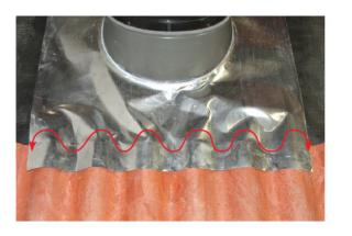
Form the bottom of the tile flashing to conform to the tile profile.
