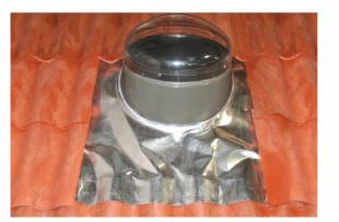
Some codes require that the dome be raised off the plane of the roof. These requirements can be met by purchasing a ZTA turret. VELUX offers a 6.5" or a 9" turret system.
