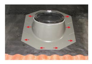
Secure the standard VELUX SUN TUNNEL™ skylight flashing to the roof deck with the screws provided.
